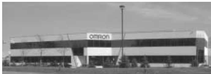
Omron Dualtec plant in Oakville, Ontario.
